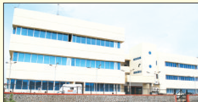
The CFS' administration building
